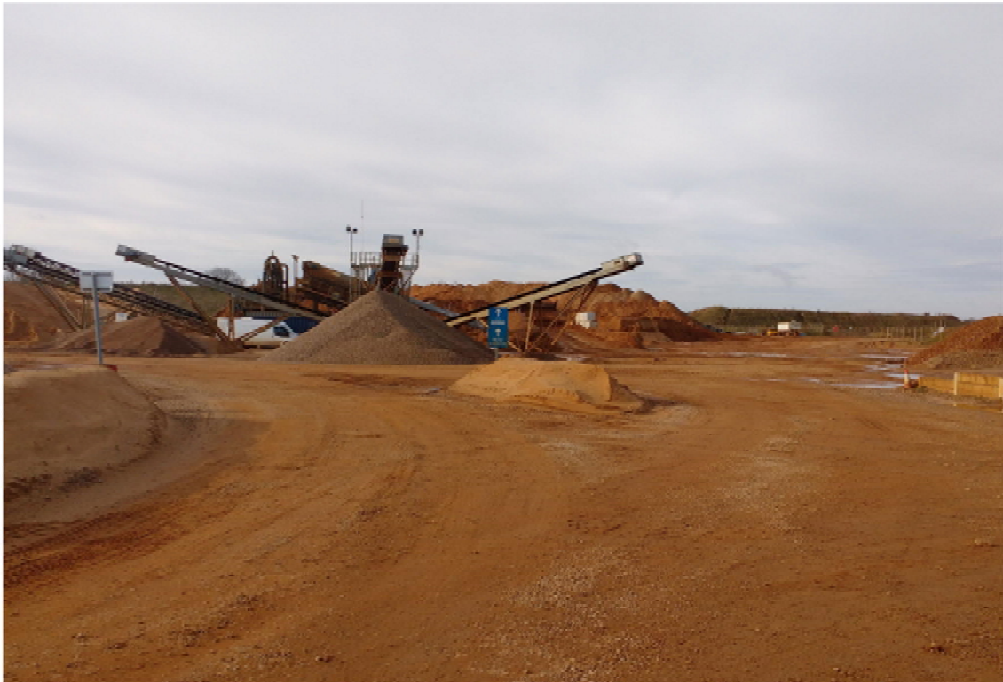
View of the processing plant at Stanninghall Quarry
